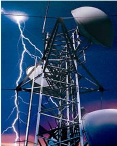
Telecoms lightning strike protection
